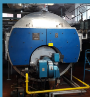
Danks 8000lb/hr steam boiler
