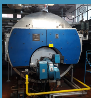
Danks 8000lb/hr steam boiler
